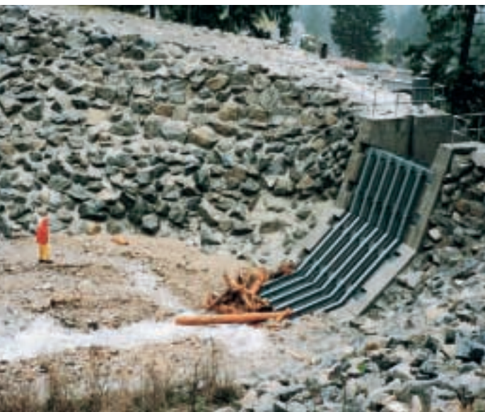
Large scale debris flow mitigation structures in southern BC include this debris basin at Mackay Creek in North Vancouver (photo: M Jakob).
